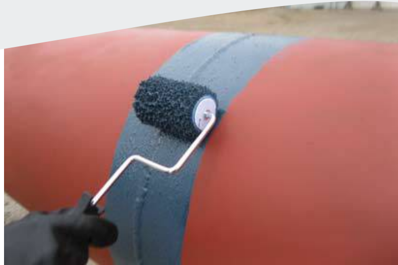
EON 1000-GP can be applied with a brush, roller or applicator pad.
