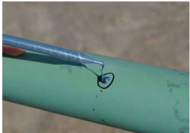
EON 1000-GP in a 50 ml cartridge used with a self mixing nozzle and 50 ml application gun for quick and effective holiday repairs.
