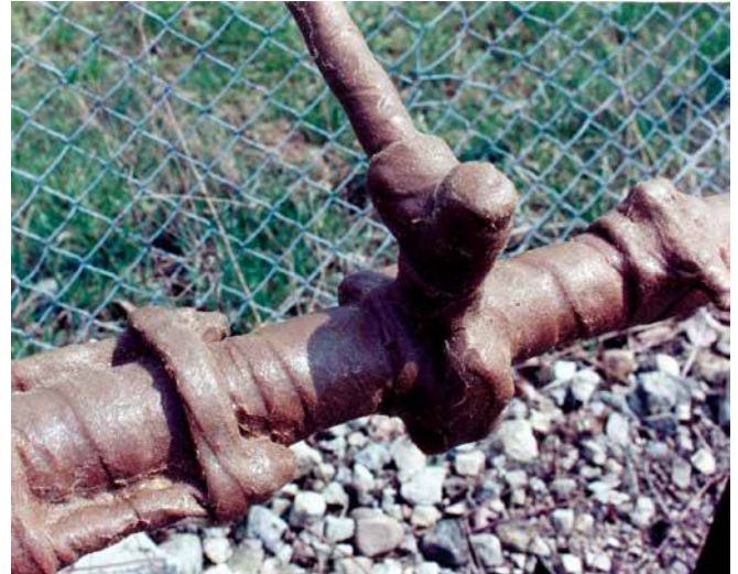
#1 Wax-Tape applied to coupling, street tee and leak clamp.
