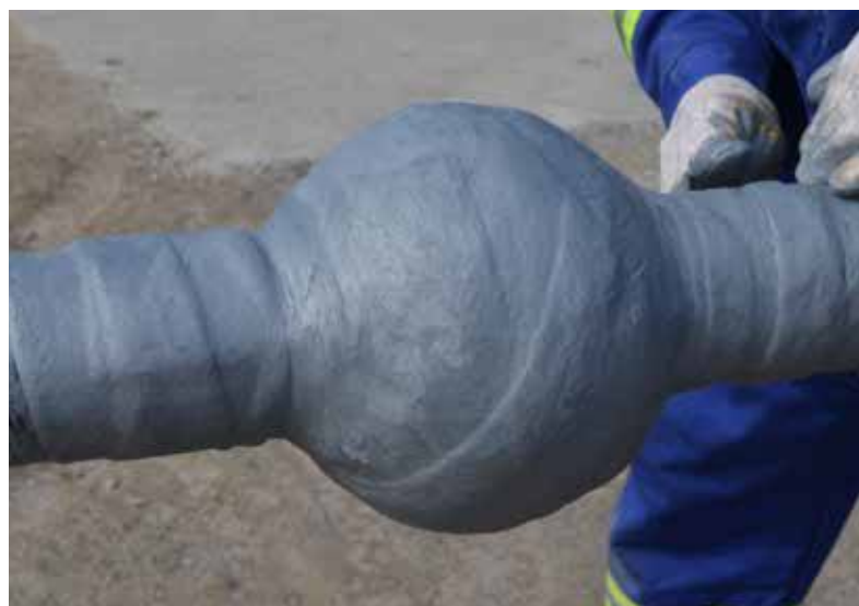
Use of Profiling Mastic creates a uniform profile for the application of Wax-Tape.
