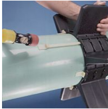
7B. Re-insert Slide-Locks completely into segment by lightly tapping Slide-Lock back into position while holding the Slide-Lock against pipe.
