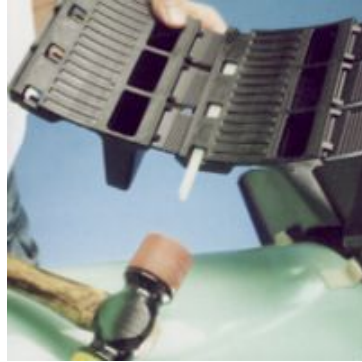
7B. Re-insert Slide-Locks completely into segment by lightly tapping Slide-Lock back into position while holding the Slide-Lock against pipe.
