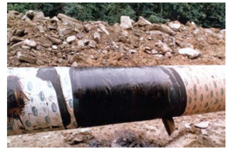
Finished application of Innercoat wax overwrapped with Guard-Wrap wrapper.
