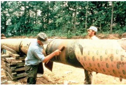
Pipe surface is wire brushed to remove loose scale, rust and dirt.
