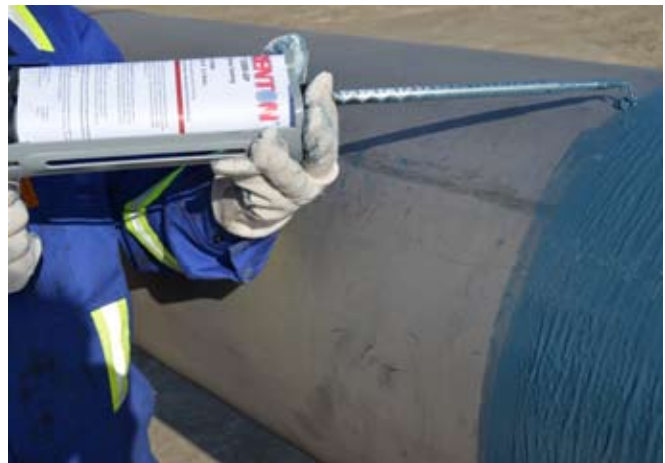
450 ml cartridge, used with the manual application gun and self mixing nozzle, eliminates mixing steps and minimizes product waste.
