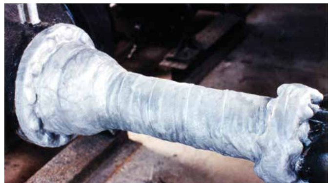
Sweating meter run pipe protected with #2A Wax-Tape.
