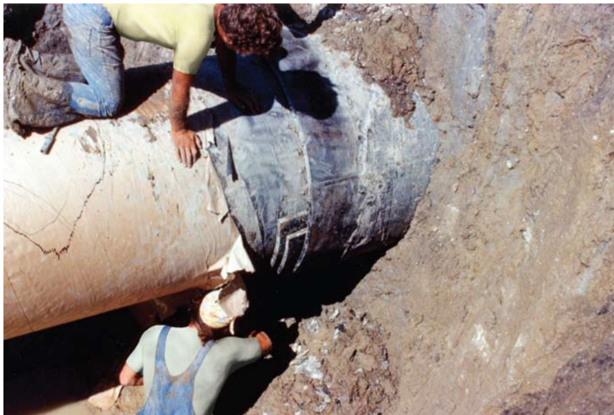
Short-Stop is an easy-to-install neoprene insulator with no metal parts. It is cut to fit any size casing.
