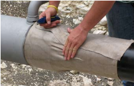
One wrap of Seal-Wrap around the casing end.
