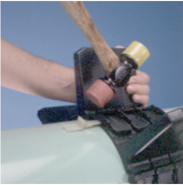
7A. To tighten Ranger II securely to carrier pipe, back Slide-Lock completely out of the slot. If needed, push segments together by hand.
