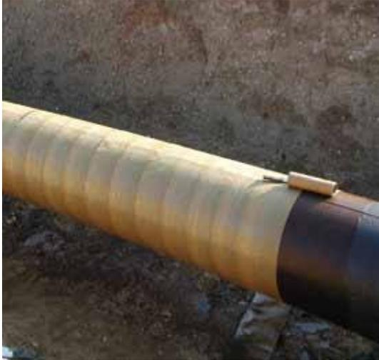
The combination of Innercoat® hot-applied wax and Guard-Wrap™ is used to prevent corrosion of belowground metal structures.
