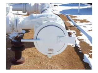
Our Yale<sup>™</sup> Y-2000 is a clamp-style closure designed specifically for 6" through 24" pipeline applications. The operation is simple, safe, does not require special tools, and does not place the operator in harm's way during any step of the opening process. Our standard design codes are ASME B31.4 and B31.8.
