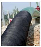
MC Outerwrap<sup>™</sup> is a specialized blend of quick curing resins impregnated into a fiberglass fabric. It provides soil stress and backfill protection to coatings that need additional mechanical strength. MC Outerwrap is specifically designed as a "hard shell" outerwrap over the Wax-Tapes. It can also be used over other coatings. It is sold complete with gloves and Trenton End Adhesive. MC Outerwrap is hand applied, with no other application materials needed.
