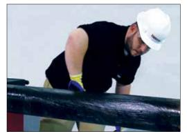
Available in brown or white, Trenton's Wax-Tape Primer<sup>®</sup> is a blend of microcrystalline waxes, plasticizers, and corrosion inhibitors (no clay fillers). It has a paste-like consistency and is designed to displace moisture and wet the surface, ensuring adhesion of the tape. This primer is typically used below ground as a surface conditioner on metal surfaces prior to using Trenton Wax Tape.
