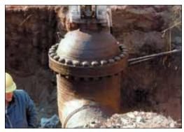
Trenton's #1 Wax-Tape® for below ground use, provides longlasting protection and is compatible with many types of materials such as steel, ductile iron and PVC.
